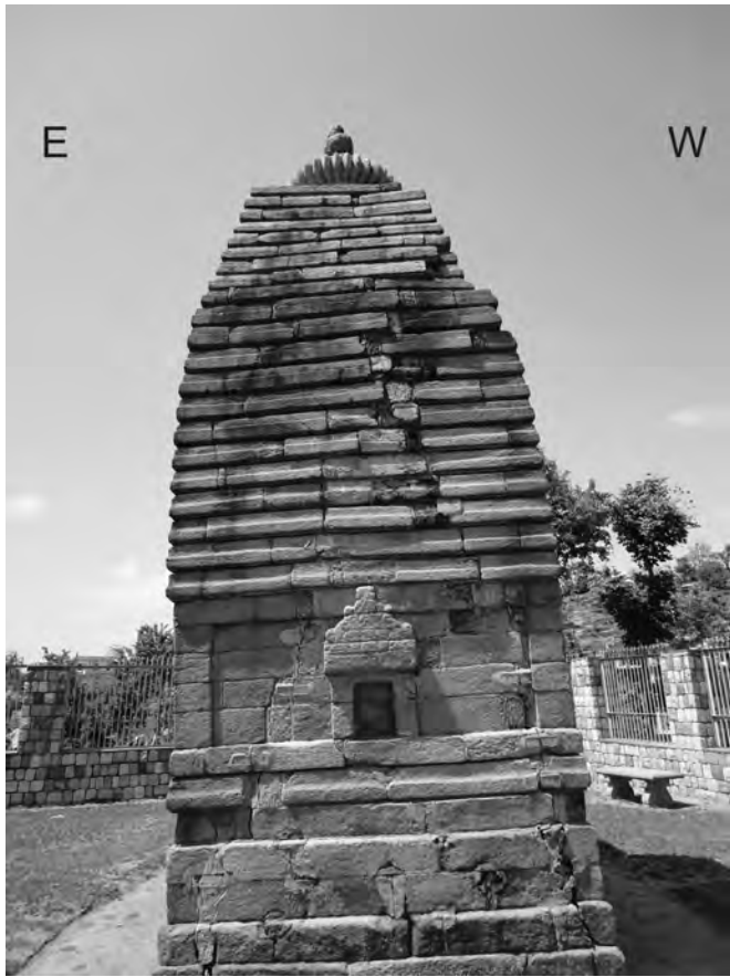
▲ Figure 5. View of Vandev temple at Dwarahat, twisted about its axis.
