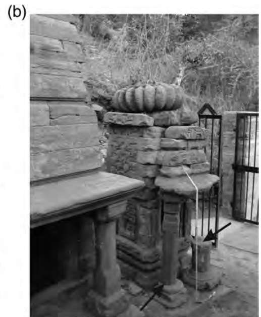
▲ Figure 6. (a) View of Katarmal temple and (b) a rotated and damaged pillar of one of the subsidiary smaller temples.
